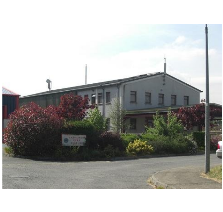
Transmitter Site Photo
